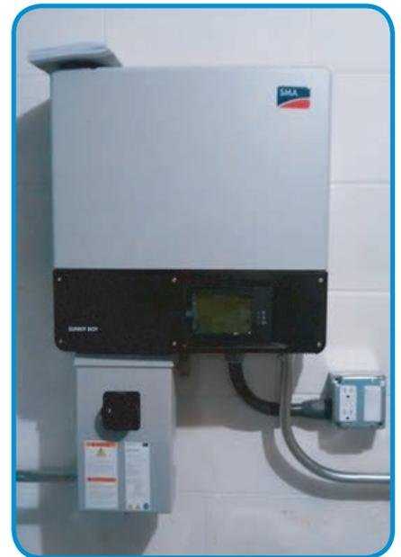
Example above of a Solar Inverter Equipped with a Secure Power Source
